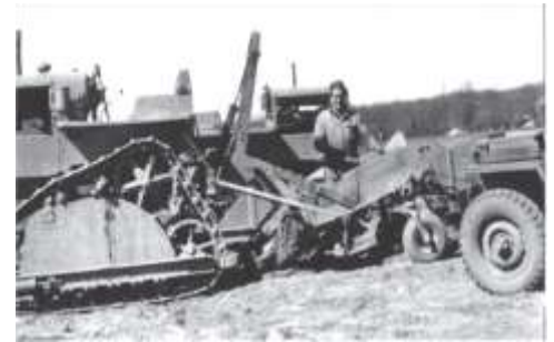
Machine modified by Princeton Nurseries for shrub digging
